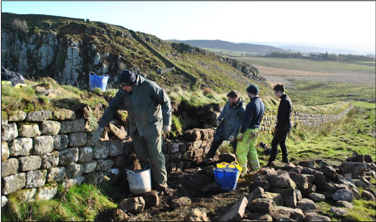
Fig.10: rebuilding at Peel Gap, west slope, looking east
