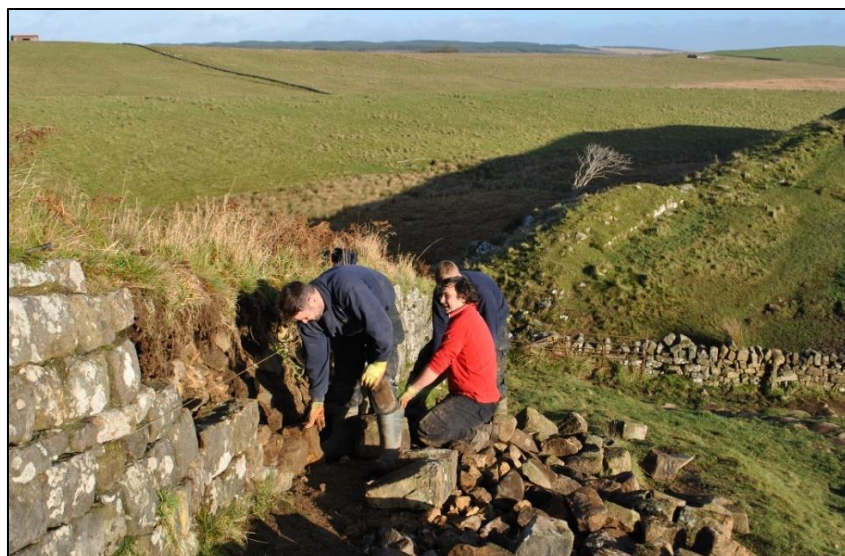
Fig. 4: Cat Stairs under reconstruction
