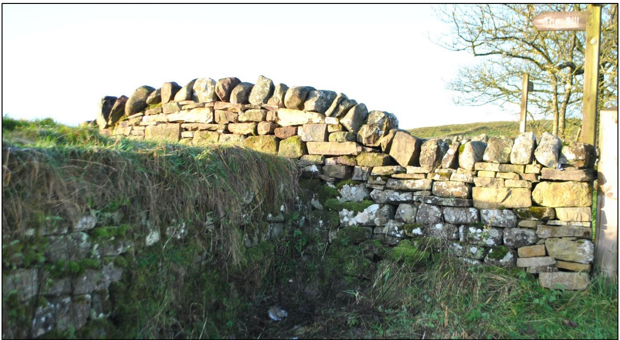
Fig. 9: raised and re-shaped stone field wall, looking south-west
