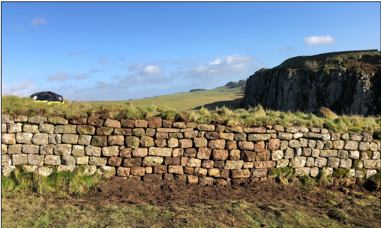
Fig. 11: Rebuilding and reprofiling complete at Peel Gap looking north-east
