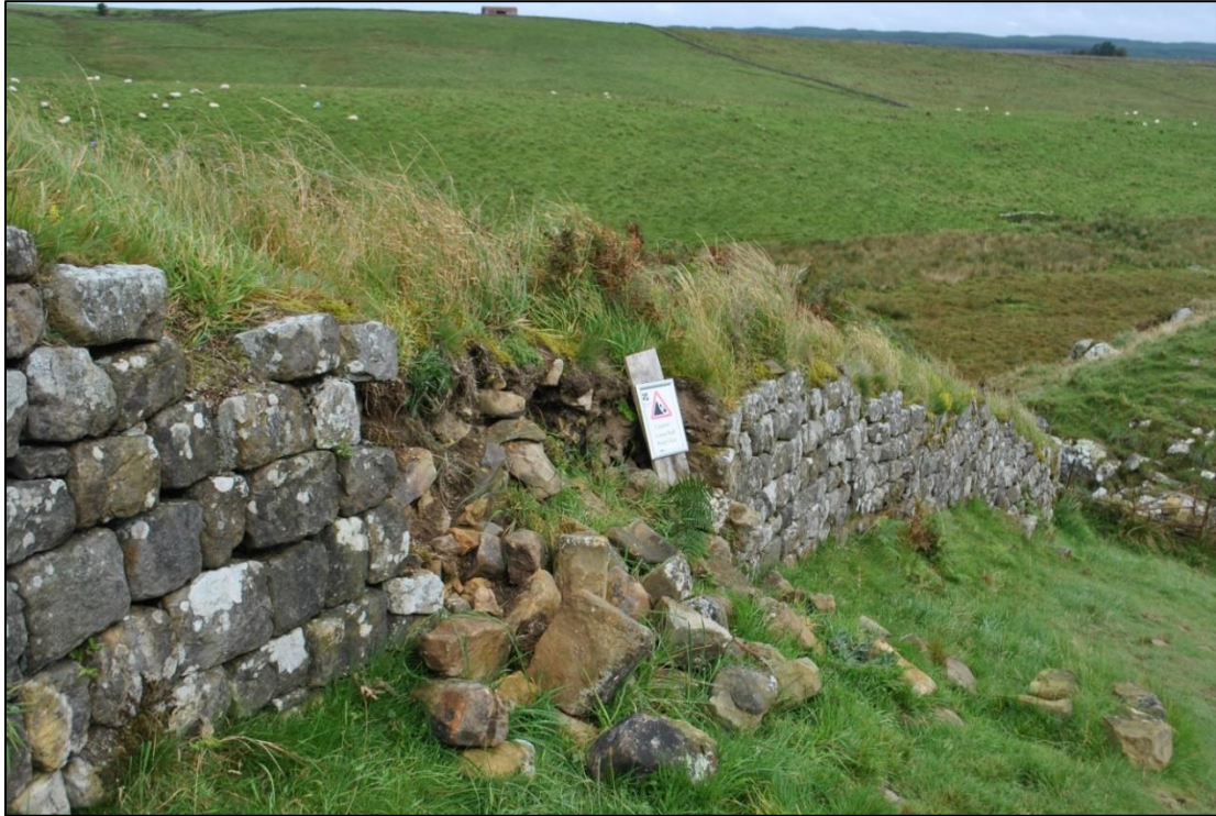
Fig. 3: the collapsed section at Cat Stairs, looking north, October 2020
