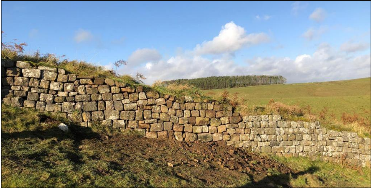
Figs 5: Cat Stairs, conservation complete, looking north-west
