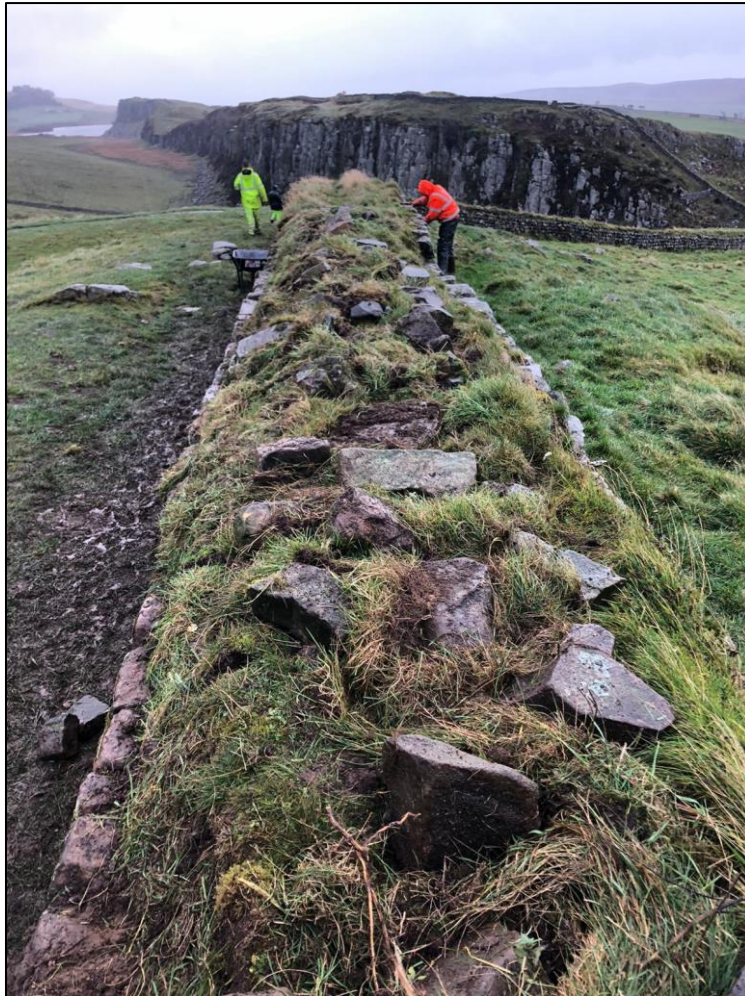
Fig. 12: Peel Gap west slope, reprofiling underway, looking east
