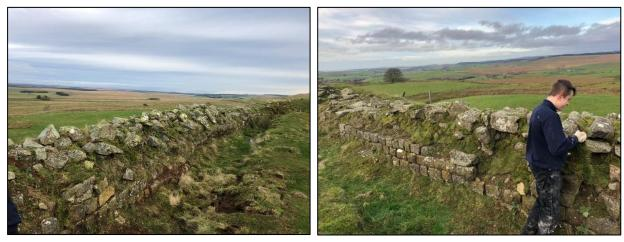
Figs 5 and 6: left, consolidated wall core looking north-east; right, consolidating the Trench 1 area
