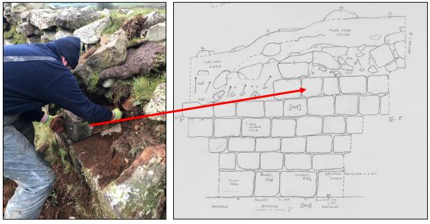
Fig. 3: left, rebedding at work in the Trench 1 area after backfilling; right, field drawing facing south showing re-set partial course and tail-bedded single stone of course above
