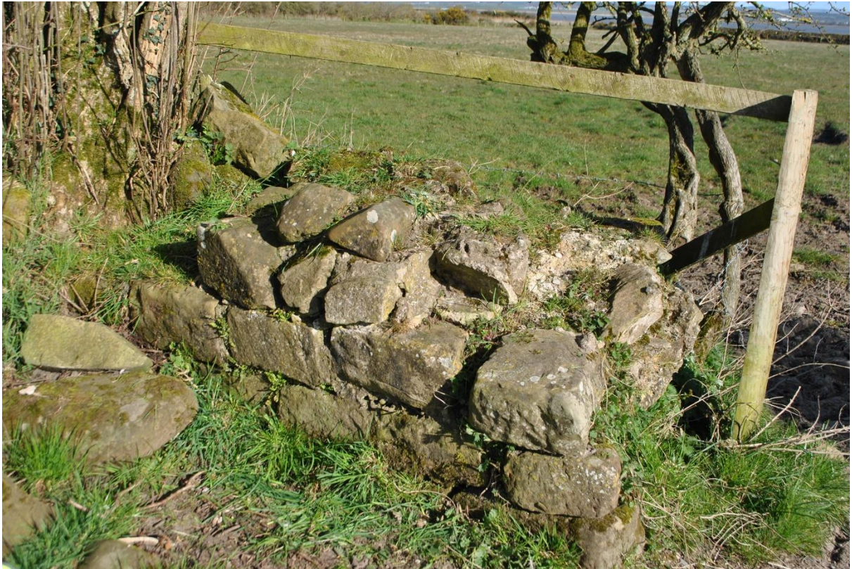
Surviving courses of the Wall west of the existing field gateway, looking north-west: April 2021
