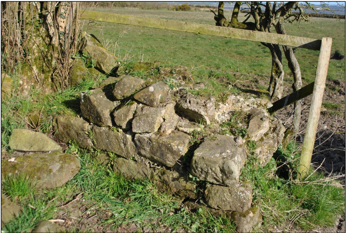
Surviving courses of the Wall west of the existing field gateway, looking north-west: April 2021
