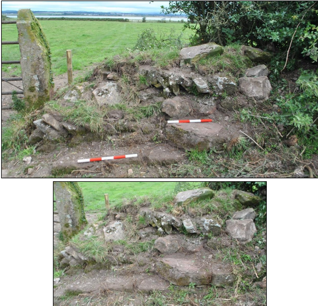
Fig. 6: East of the gate: in-situ facing stones. Lower photo shows partial upper course. Photos looking north
