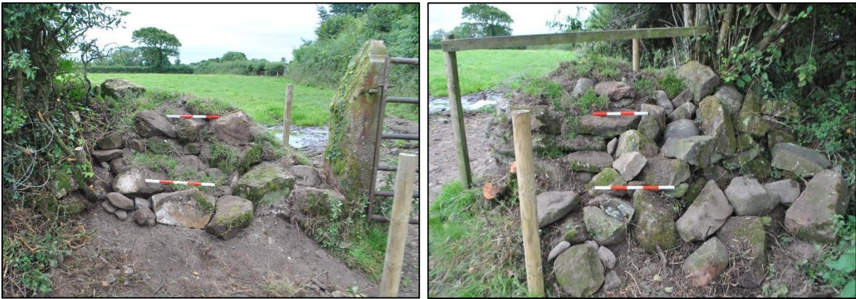
Fig. 2: re-piled loose core stones protecting the in-situ southern facing stones. Left: east of the gate; right: west of the gate. Looking south-west
