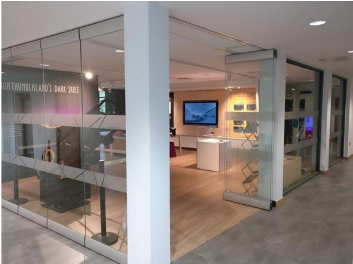
The Stell exterior showing entrance and glass wall panels on the left and fixed glass walls to the right.
